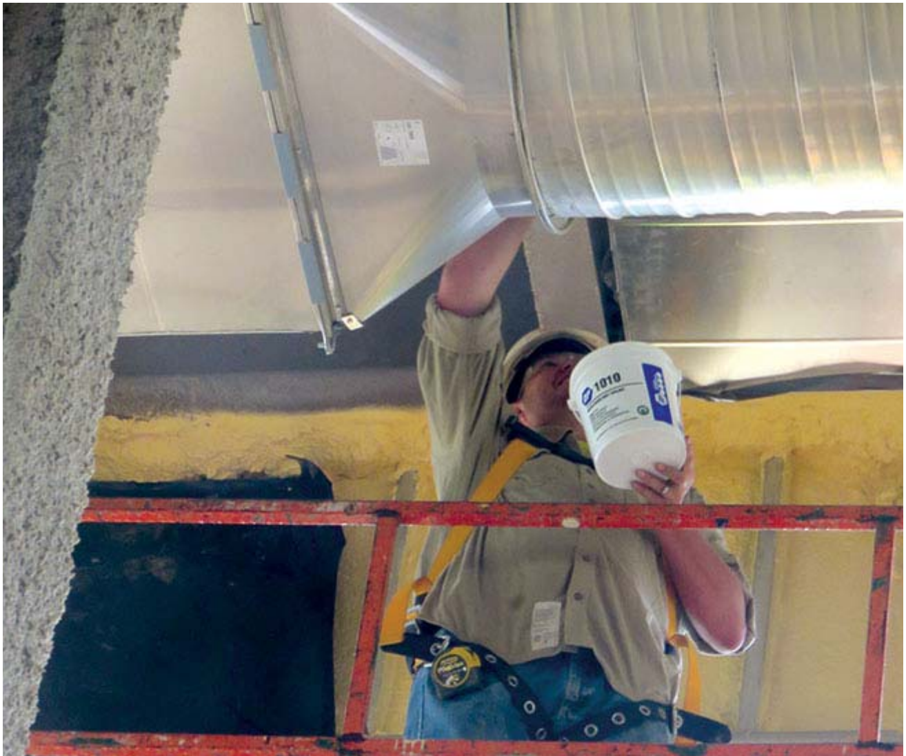
Vaughn Industries Mike Swirlain seals duct on a project in Columbus, Ohio.
